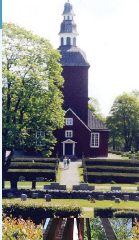
The lovely timber church that only sits on the ground
